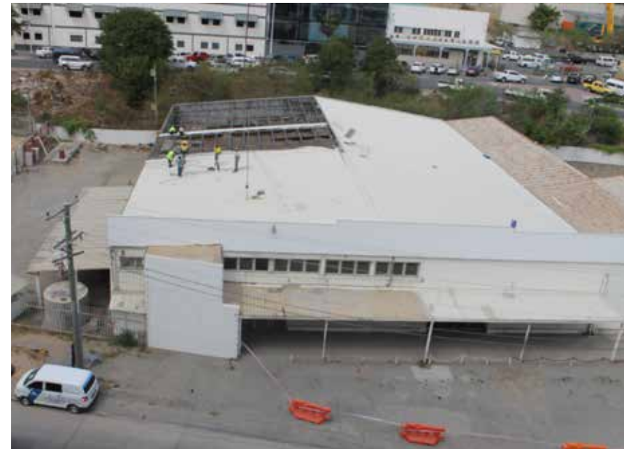
ABOVE: The site prior to demolition commencing.
