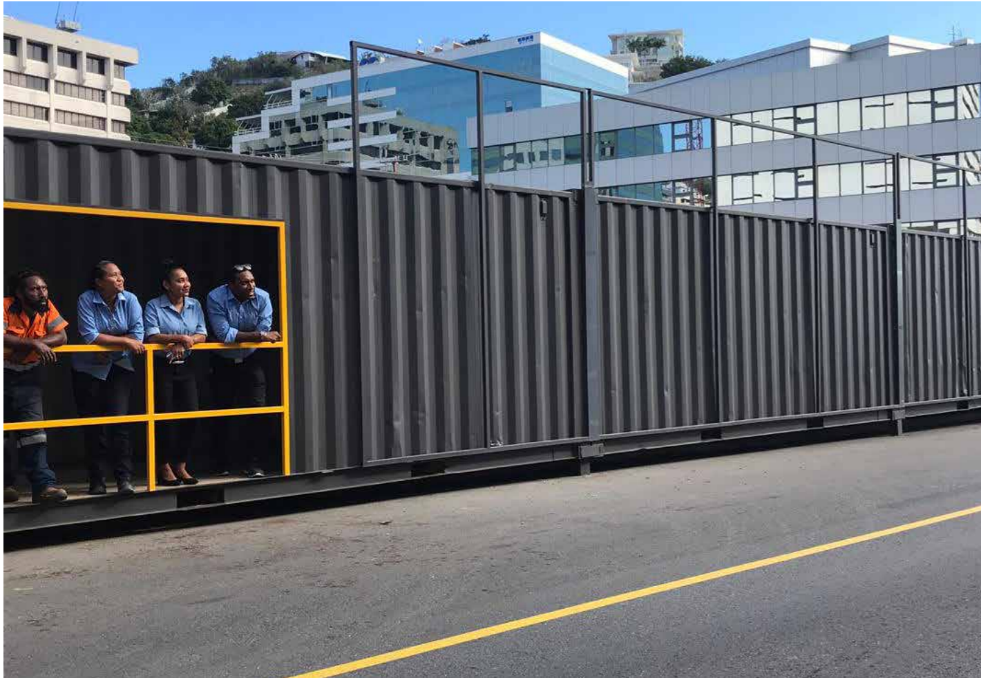
Containerised Pedestrian Safety Gantry System at Harbourside South, Port Moresby
