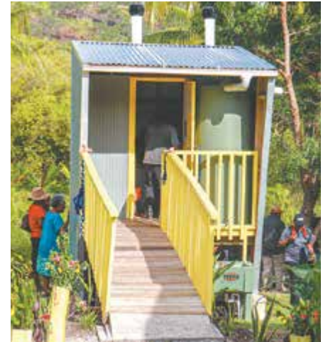
Sago dry toilet commissioned at Barakau aid post. There are nine sago dry toilets throughout the village.
